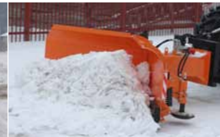
PUV 2800 model at work in Y position -pushing the snow forward
