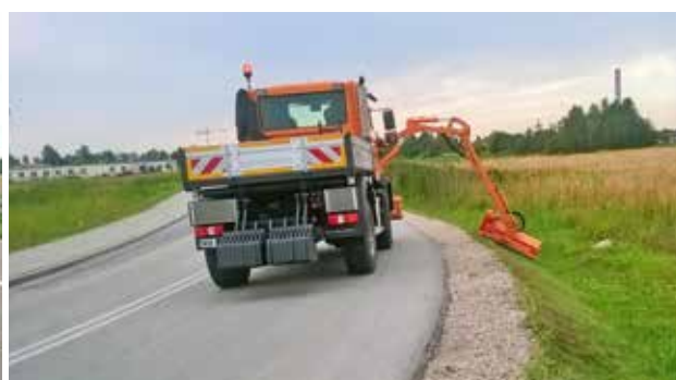
Mowing of a hard-to-reach roadside using a WWP500UH multifunction arm and GK 110 head
