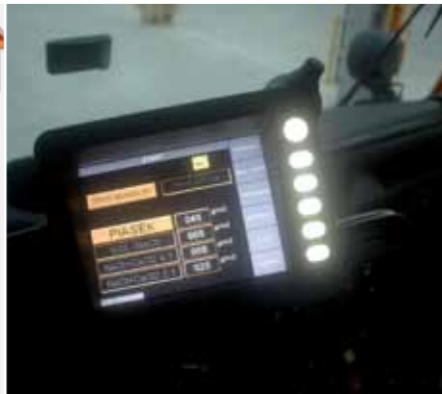
Bosch-Rexroth control panel
