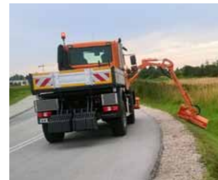
Mowing of a hard-to-reach roadside using a WWP500UH multifunction arm and GK 110 head.
