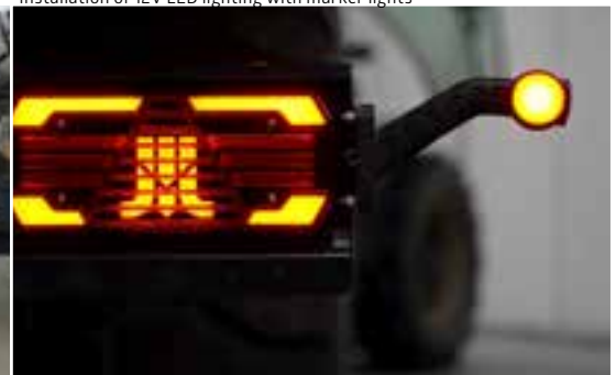
Installation of 12V LED lighting with marker lights
